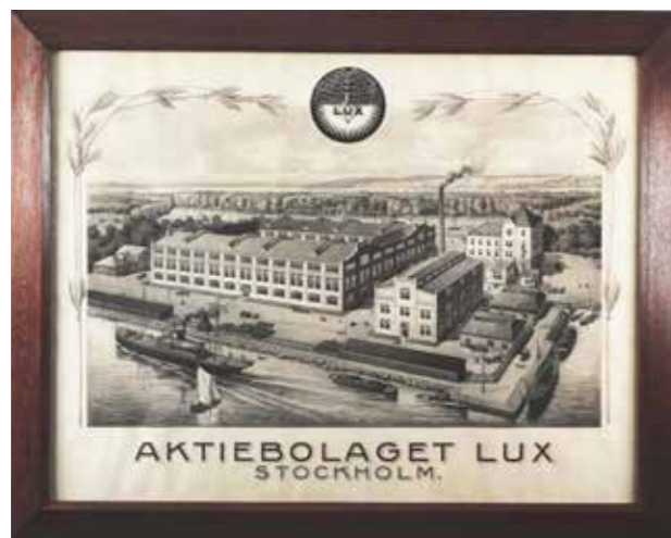
The factory on the island Lilla Essingen where Lux moved in 1908. The building furthest to the right, below the chimney, and the white house in the background are still there to this day.
