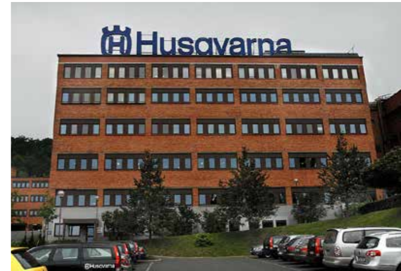
Husqvarna AB's offices and factory in Huskvarna. The company is one of Europe's oldest, founded in 1689 as a rifle factory.
