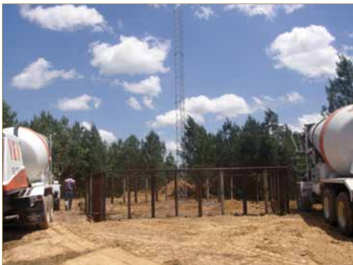
Towers under construction
