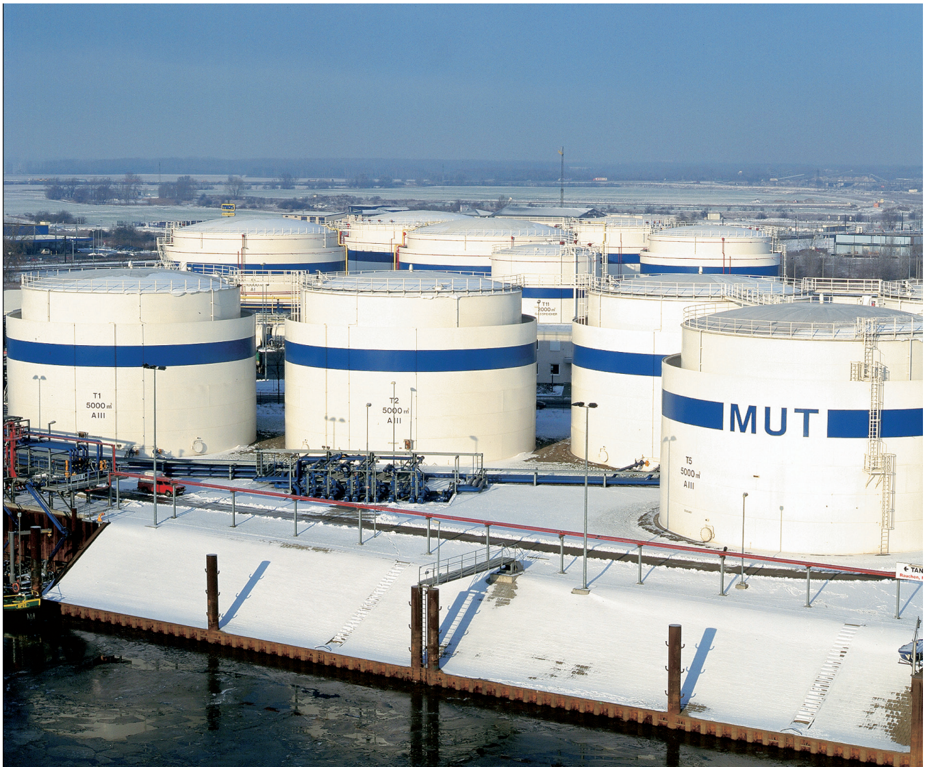
The FCU works as a data concentrator for a group of tanks ensuring fast data communication from the tanks to the control room.
