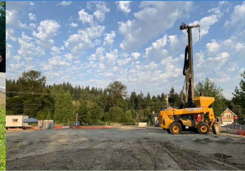
Earthwork begins at the Encompass Snoqualmie site.
