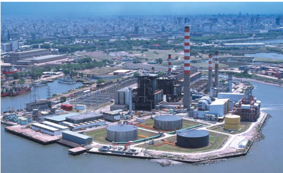
Costanera Power Station, Argentina
