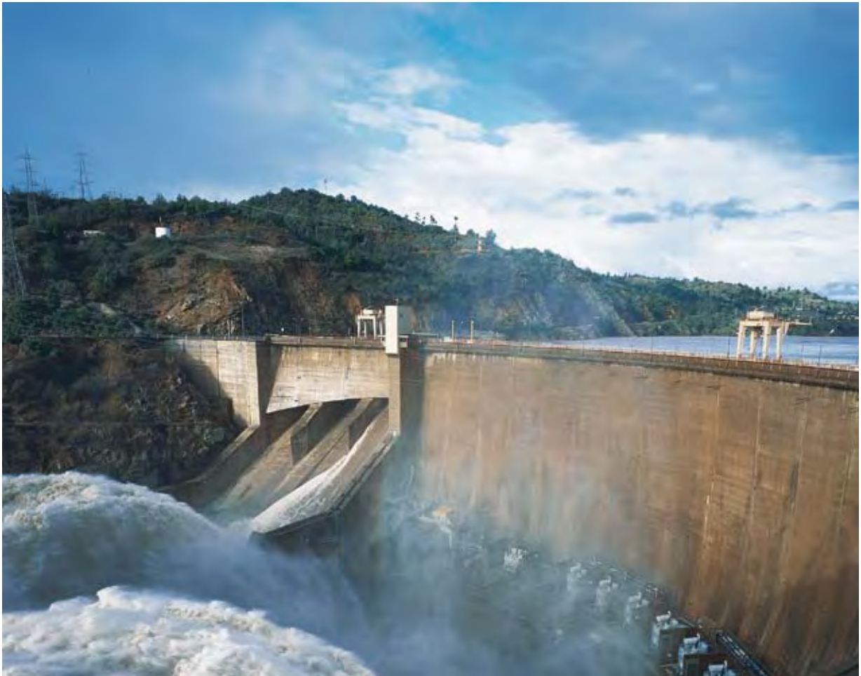
Power Plant Rapel, Chile
