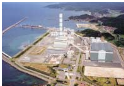
Misumi Thermal Power Station (Coal)
