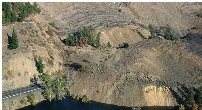
Photo of the 2009 Nile Landslide
