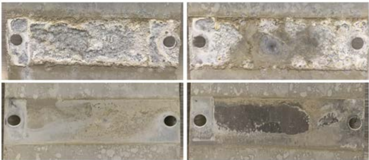
Figure II.3.I.7. Corrosion of AA6022 baseplate exposed to nine weeks of R-343 full vehicle corrosion testing. Note the extensive corrosion of the baseplate under both CFRP top plates. Corrosion was higher for AA6022-CFRP Random. AA6022-AA6022 shows signs of dirt accumulation and AA6022-fiberglass shows signs of bare metal. Source: Ford.
