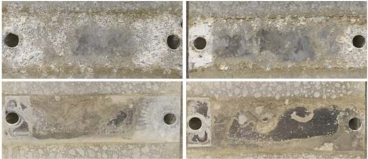
Figure II.3.I.6. Corrosion of AA6111 baseplate exposed to nine weeks of R-343 full vehicle corrosion testing. Note the extensive corrosion of the baseplate under both CFRP top plates (higher for AA6111-CFRP Random). AA6111-AA6111 and AA6111-fiberglass coupons show signs of bare shiny metal with traces of dirt. Source: Ford.
