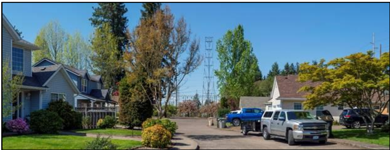
Photograph 3-29. View of the communications structure within the BPA Albany Substation from the residential neighborhood on Orchard Lane (KVA 14), looking west.
