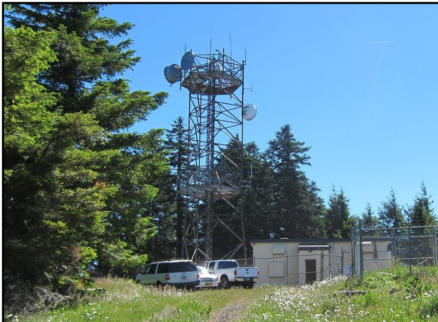
Photograph 2-14. CPI West Point Spur communications site, facing east.
