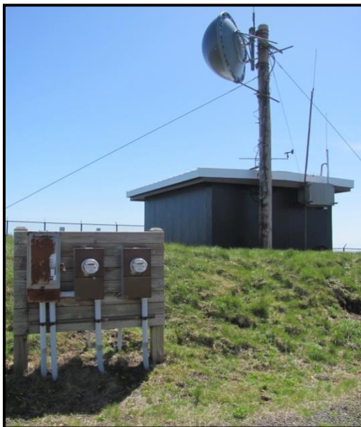
Photograph 2-7 (left). The electrical station service pedestal with BPA and USFS meters.
