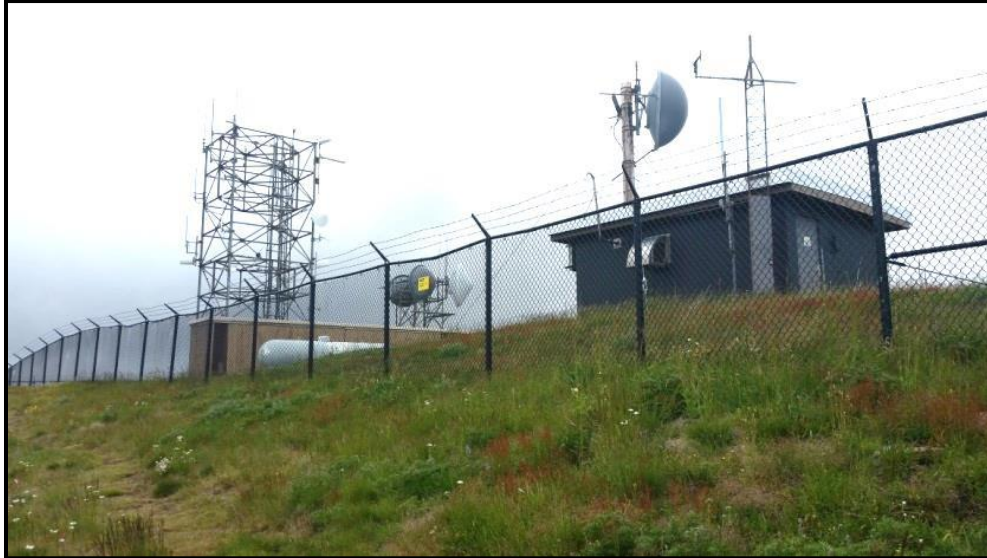
Photograph 2-6. Marys Peak communications site, looking west.
