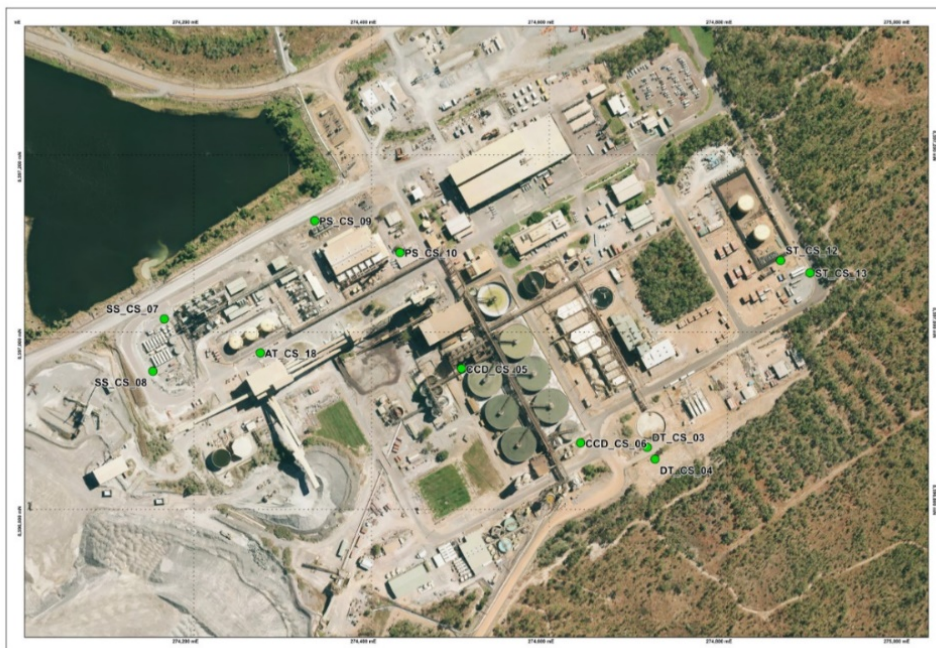
Figure 5-94: Locations of soil bores drilled in the processing area at Ranger Mine
