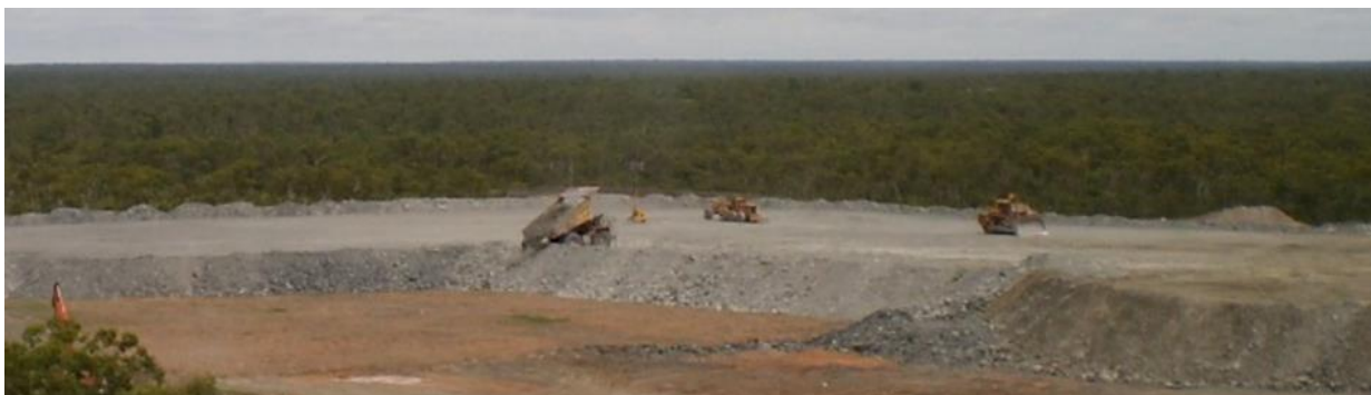
Figure 4-26: Tip head dumping of the lower layer(s) during TLF construction
