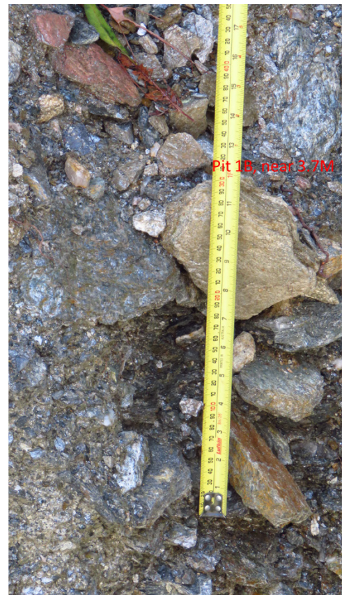
Figure 4-19: Presence of roots of 1-2 mm in diameter visible at 3.0 m deep in the Pit 1A and at 3.7 m deep in the pit 1B of the TLF
