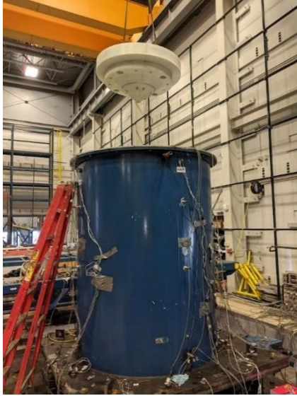
a. positioning the plug using an overhead crane
