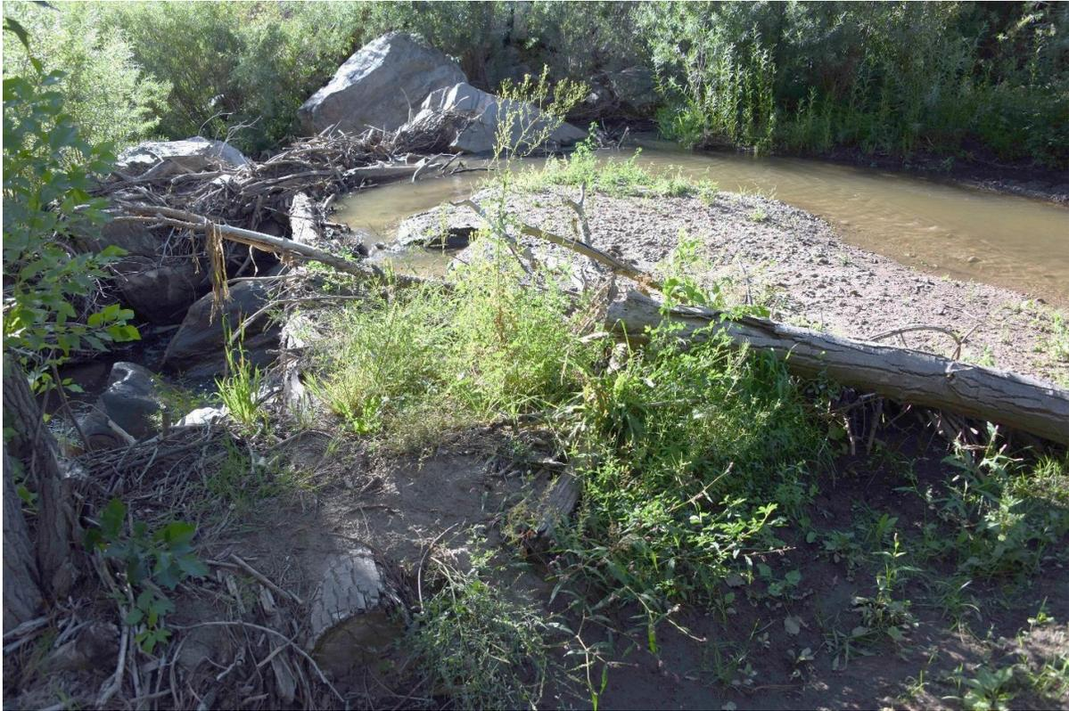
**Figure A13b. Artificial stabilization with one-log dam that is capturing sediment and creating a new gravel bar and sediment sheet in the channel.**
