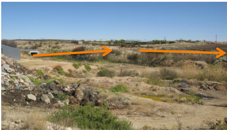
Photo 12: The section of the proposed pipeline, crossing underneath the N14 (through an existing culvert) and then running next to the seasonal stream towards Picture 11).
