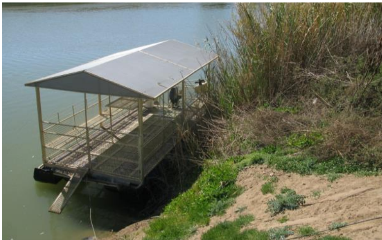
Photo 6: The banks of the Orange River at the proposed pump station location (looking from the disturbed area eastwards).
