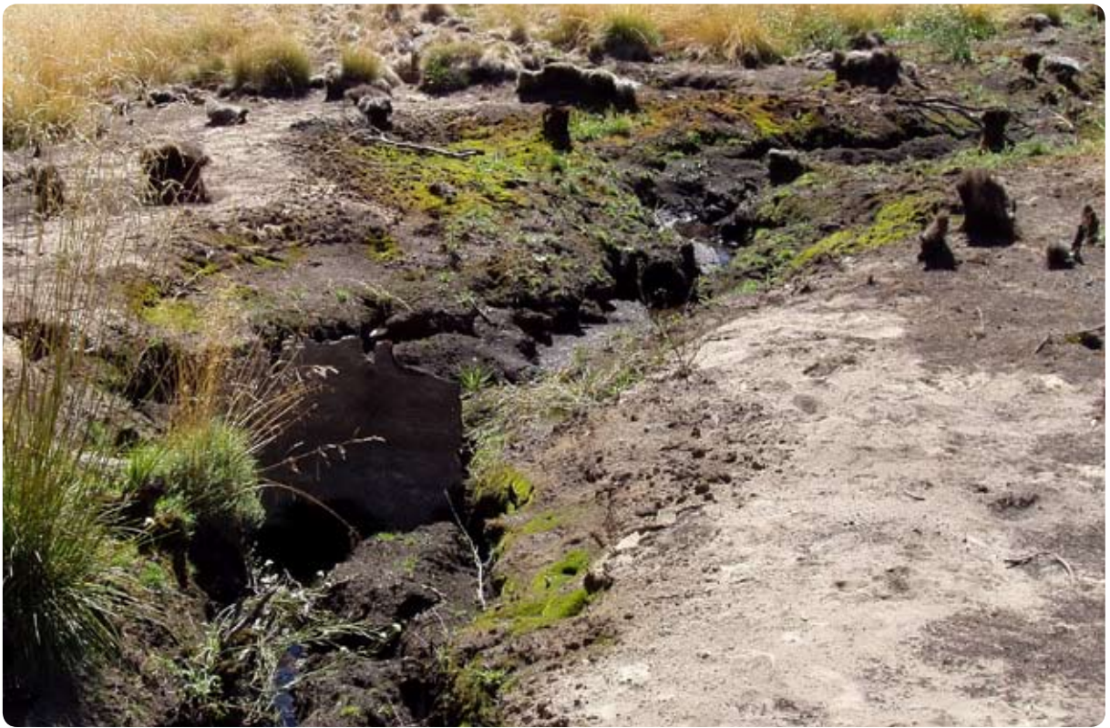
Figure 18: Peat fire damage at Top Flat showing bank collapse in 2004. The partially burnt board is a barrier placed after the 1983 fire
