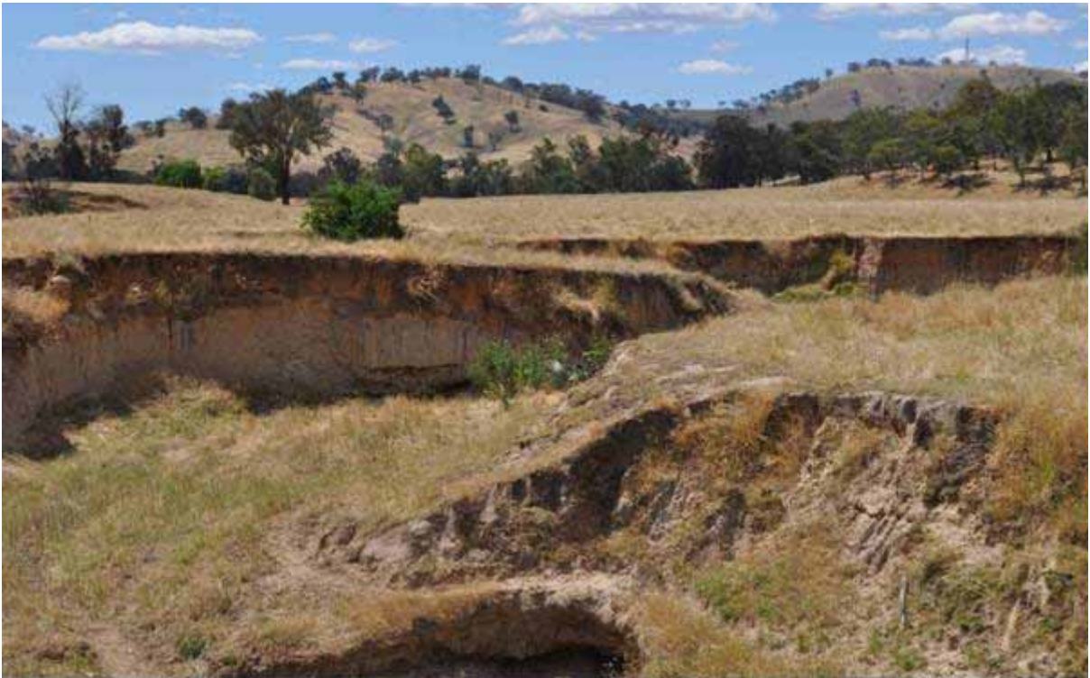
Photograph 5a. Drainage plain with highly concentrated run-on, sodic subsoils and gully erosion
