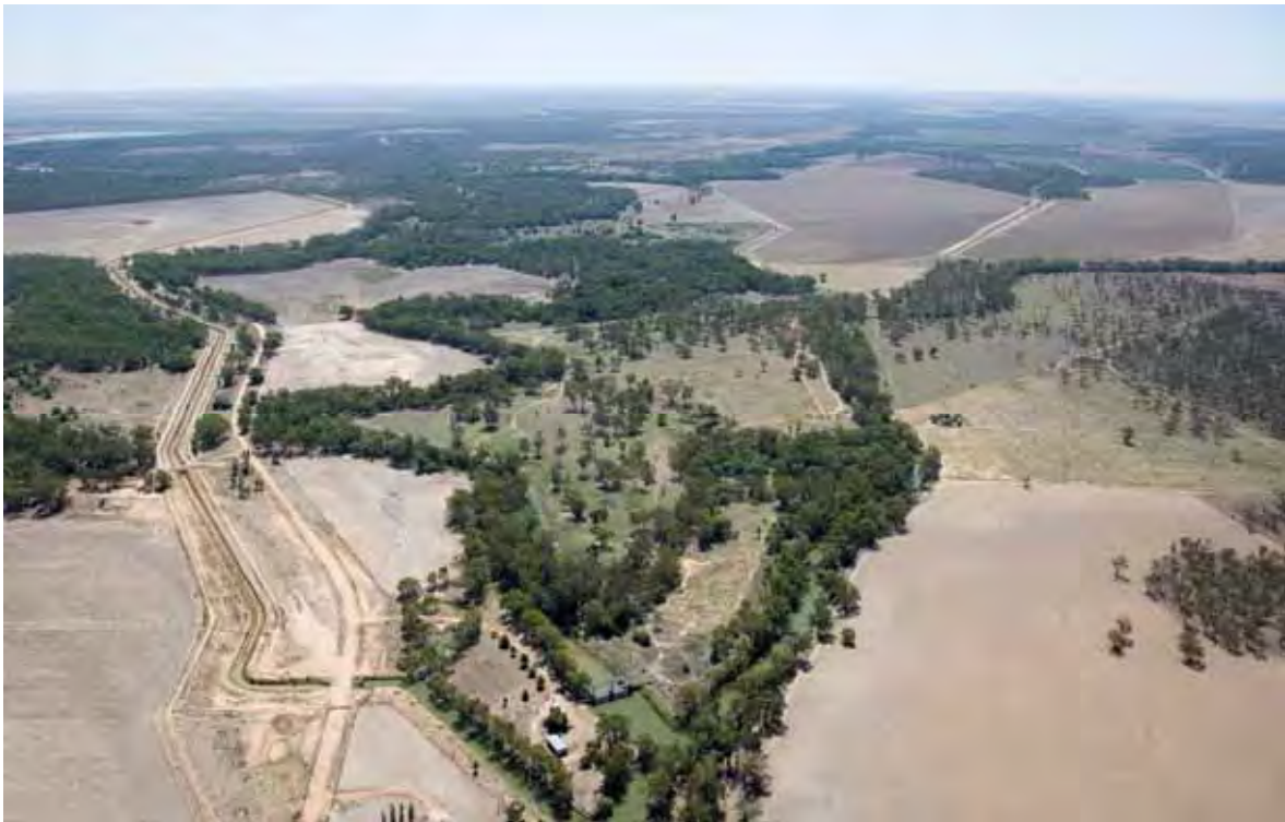
Photograph 3: View downstream at Marebone Weir. Irrigation supply channel on left, Macquarie River centre, and Marebone Break on right (Photo: Grenville Turner, 2007)
