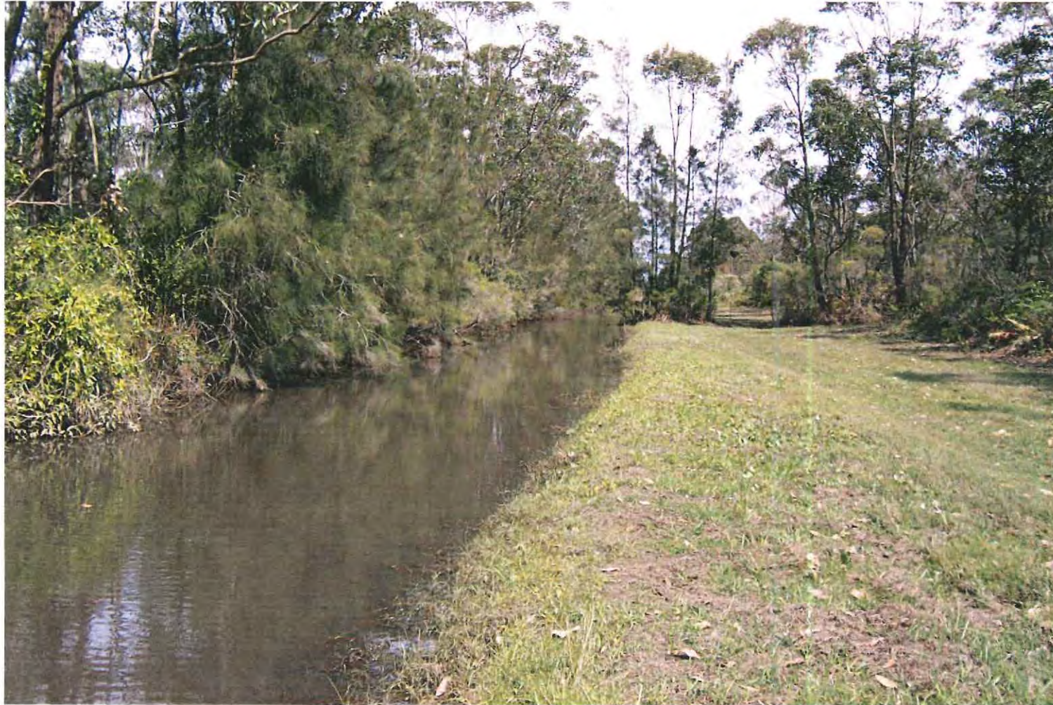
Figure 4 – Unrestricted flow situation in the middle reaches of Campvale drain
