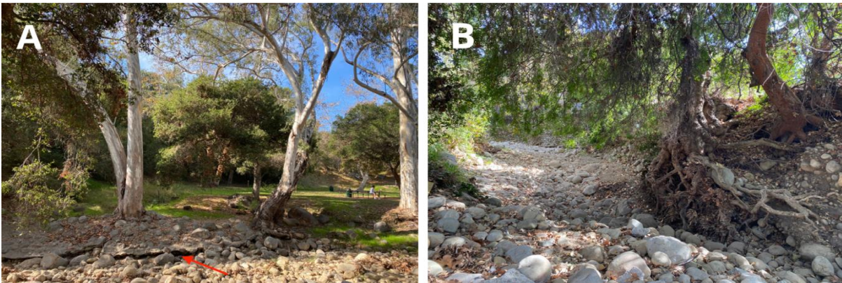
Figure 31A. Three large eucalyptus trees on the west bank of Mission Creek in Oak Park. Concrete embankment indicated by the red arrow. Figure 31B. Mission Creek bank stabilized by sycamore tree roots. Blackwelder. 2021.
