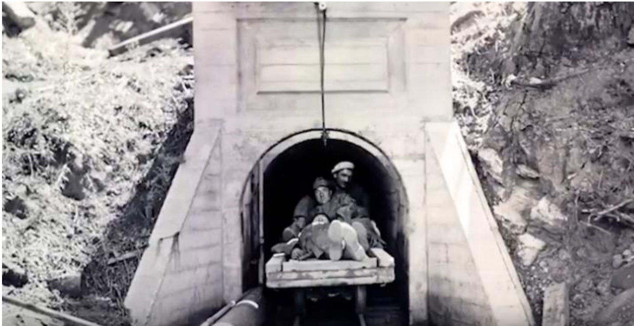
Figure 24. Workers inspecting Mission Tunnel. Unknown photographer. From EdHat. February 26, 2019.
