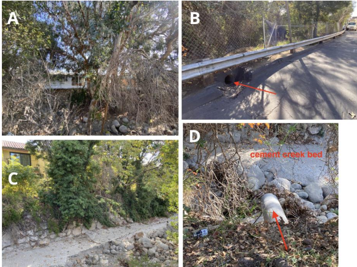
Figure 27A. Mobile home hanging over the Eastern bank of Mission Creek. The large eucalyptus tree is providing support as it is rooted into the bank. Figure 27B. Unfiltered storm drain from the parking lot of Presto Pasta and Grocery Outlet, is leading straight into Mission Creek. Figures 27C and 27D. Cemented bed and bank of Mission Creek. Blackwelder. 2021.
