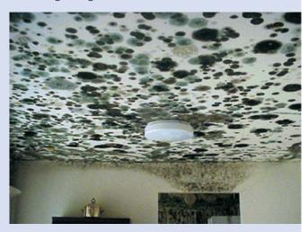
Photo 2: Extensive mold contamination of ceiling and walls
