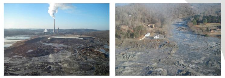
Figure 3. Remaining ash in cell where the breach occurred in 2008 (left). Flow of ash into the Emory River from the breach (right). (*Source*: EPA)
