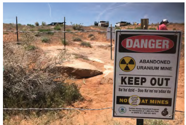
Figure 1: Cyprus Amax closed and fenced this mine opening at the Plot 6 mine in Tse Tah. This interim action was taken to address physical hazards while the full extent of contamination at the mine is assessed
