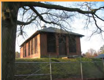
Photograph 2-3: Aerator Building Looking from the North
