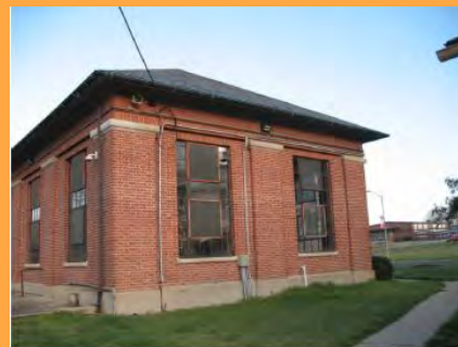
Photograph 2-1: Pump Building Looking from the East
