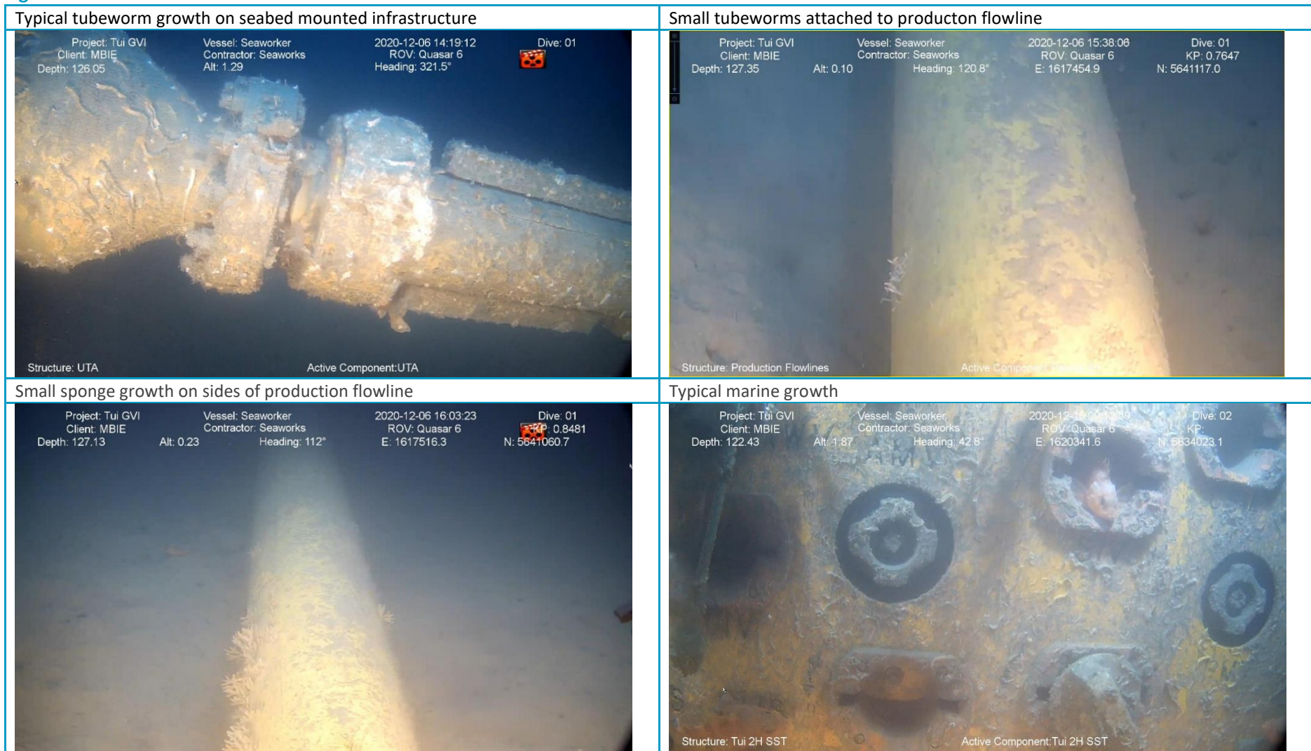
Figure 8 Marine Growth Observed on and Around Seabed Mounted Subsea Infrastructure
