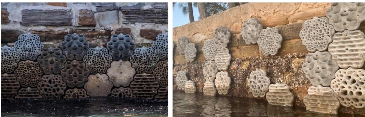
Figure 50: Examples of retrofitted living seawalls.
