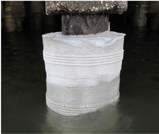
Figure 51: Example of EConcrete pile sleeve
