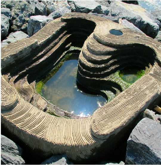
Figure 52: Example of EConcrete constructed rock pools.
