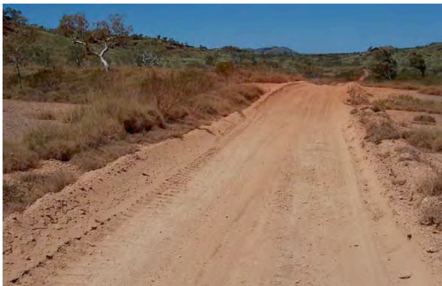
Plate 6.2: Access track through the valley containing the population of Ptilotus sp. Brockman (note lowering of track surface compared to surrounding soil level).
