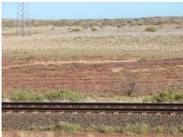
Plate 5.1: Narrow band of vegetation unit FRaHA (backed by SPOv) on western side of existing rail.
