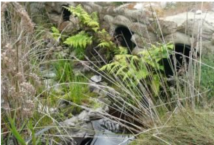
Photograph 4 - Shows the existing water crossing on the nearby Summertime Track. The crossing shows multiple culverts with concrete filled sandbags as scour protection.
