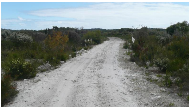
Photograph 1- shown left is of the nearby Summertime Track and provides an indication of the type of construction proposed for Doggerup Road. The limestone material is placed on top of the existing ground surface without the formation of defined roadside drains. Note is also made here regarding how the approach to water crossings are made, where an existing water crossing is located beneath the guide posts in the photograph.
