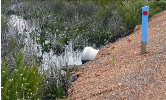
Photograph 3 - Shows an existing culvert crossing installed by the Shire of Manjimup on Windy Harbour Road. Note is made of the use of reinforced concrete pipework and the Main Roads standard guidepost as a vehicle notification of the crossing.
