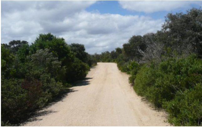
Photograph 2 - D'Entrecasteaux Road within the Windy Harbour townsite. A 3.0m wide limestone track with the vegetation regrowth occurring right up to and even overhanging the track. It should be noted that the track is constructed to take higher traffic volumes than that proposed for Doggerup Rd and has minimal track width, no defined drainage and the track elevated above natural surface level by the actual track pavement.
