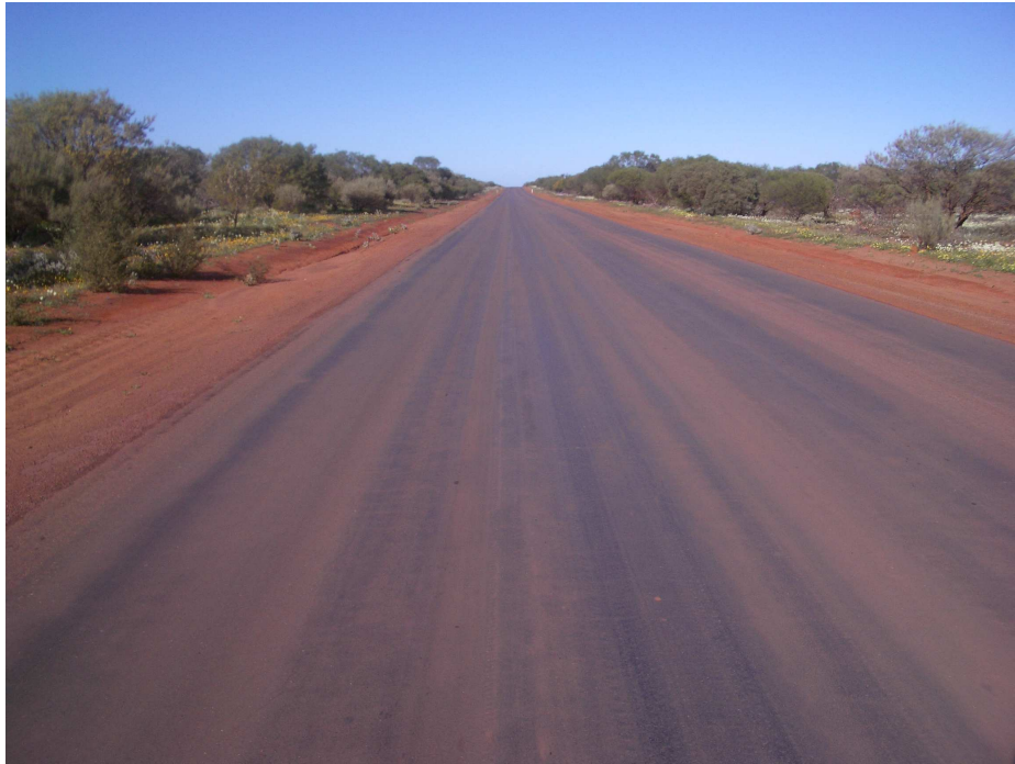
Plate 1: Bitumen Sand Seal
