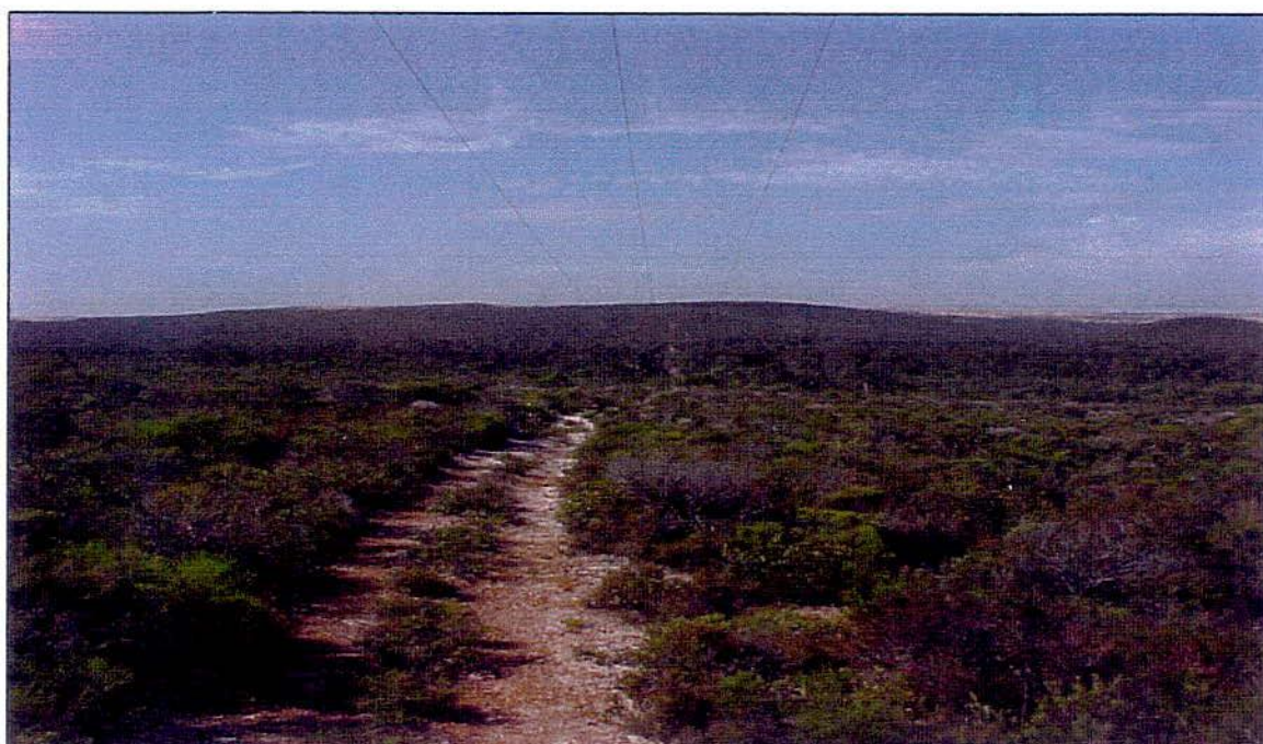
The Existing 132kV Cataby to Encabba Transmission Line Within Coomallo Nature Reserve
