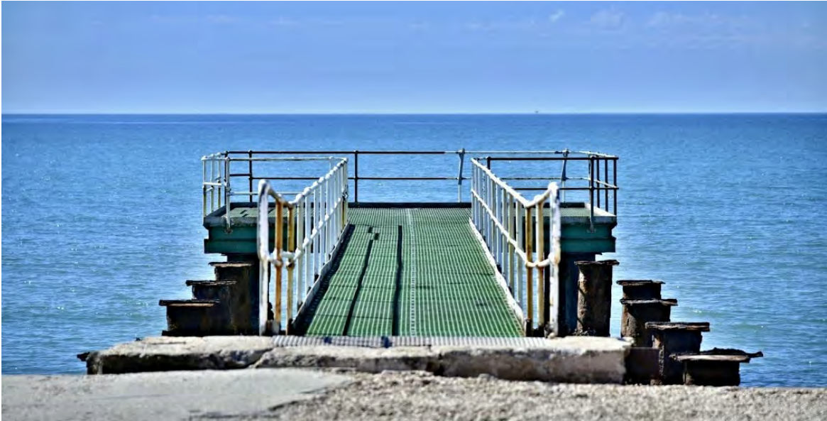
Figure 4-7: Photograph looking seaward from the base of the Learmonth Jetty abutment
