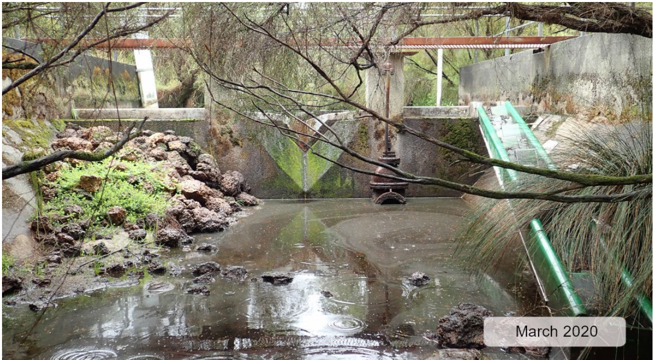
Plate 3: Walpole River Weir (downstream) (DWER 2020)
