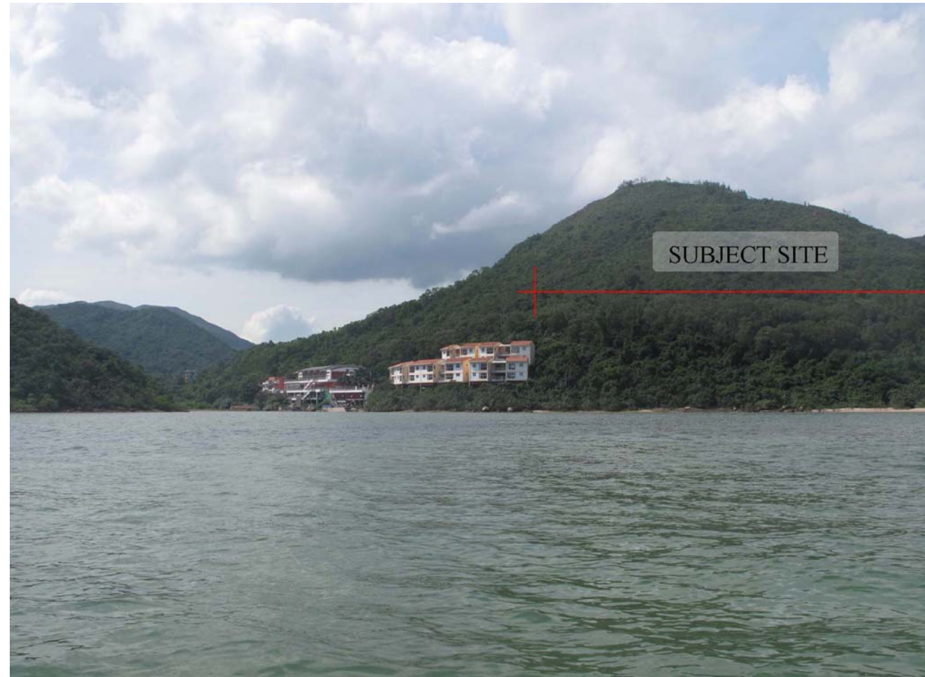
VPT 3.4 - View north from water channel between work site and Yim Tin Tsai
