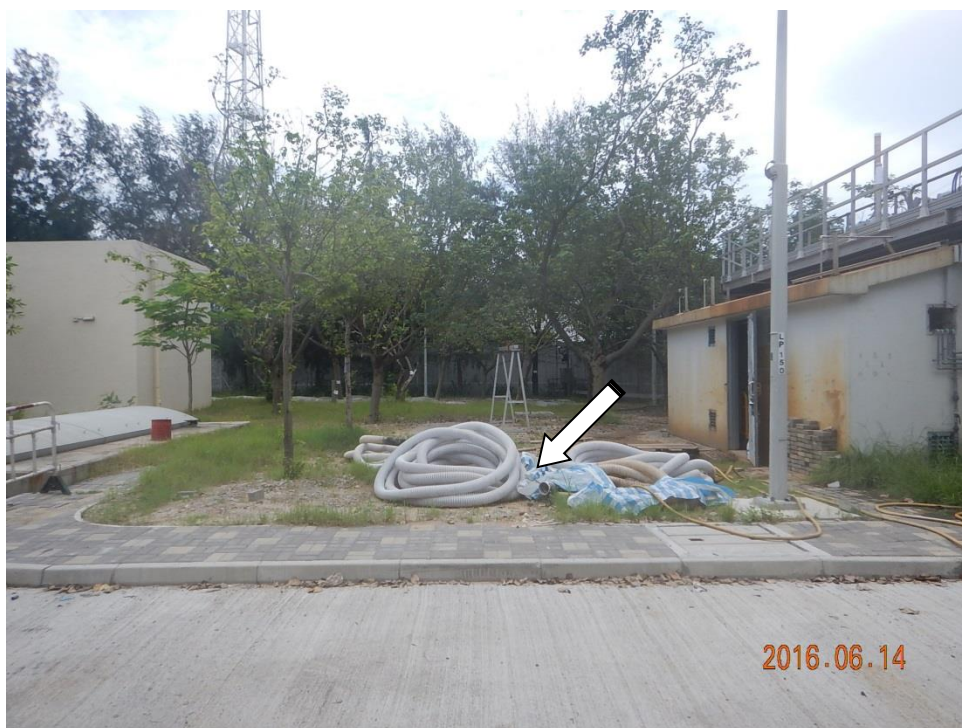
Photo no. G-19 : Groundcover and Lawn were observed missing during the site inspection.
