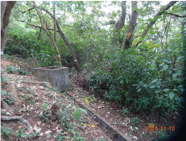
Photo 7. General View of Project Site (inside Natural Woodland)
