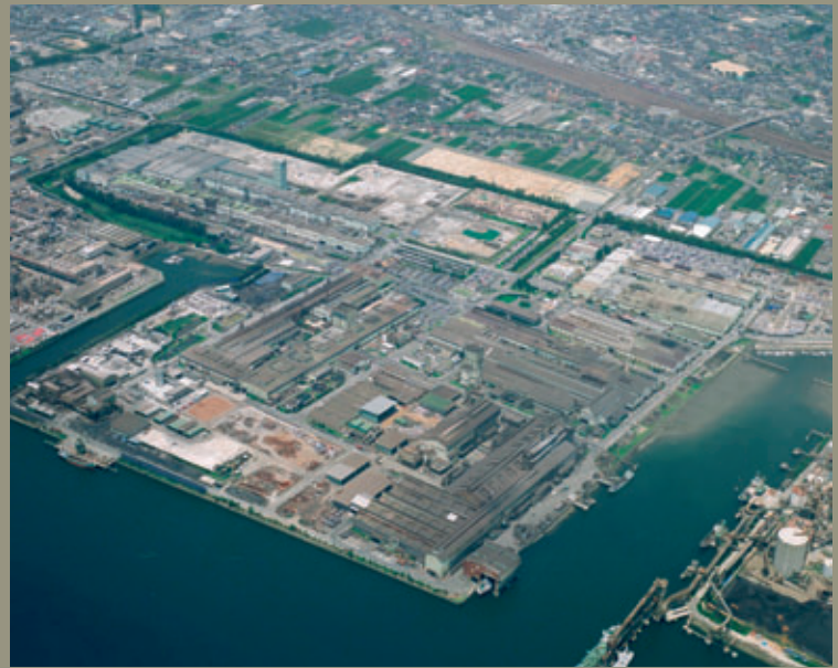
Aerial view of Nisshin Steel's Shunan, Japan plant.
