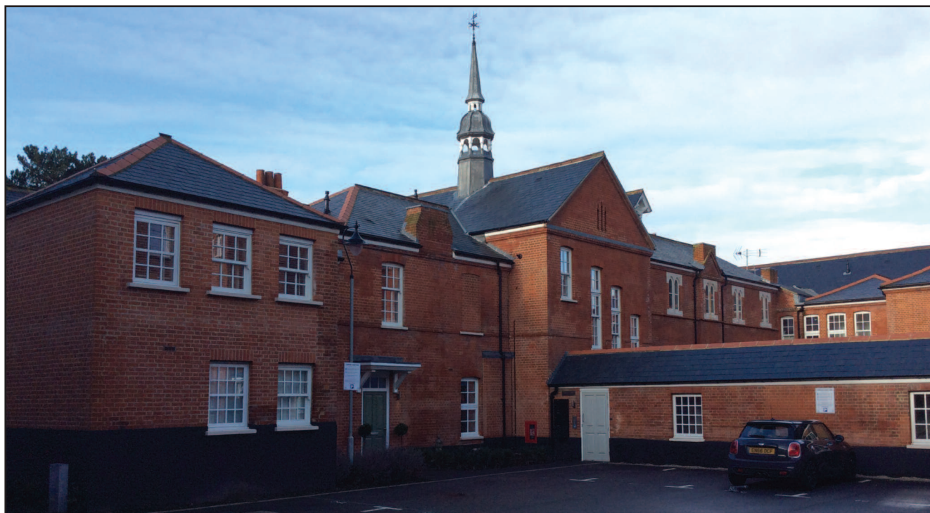
3. Back of the renovated Chelmsford Union Workhouse, 2017 (Author's photograph)
