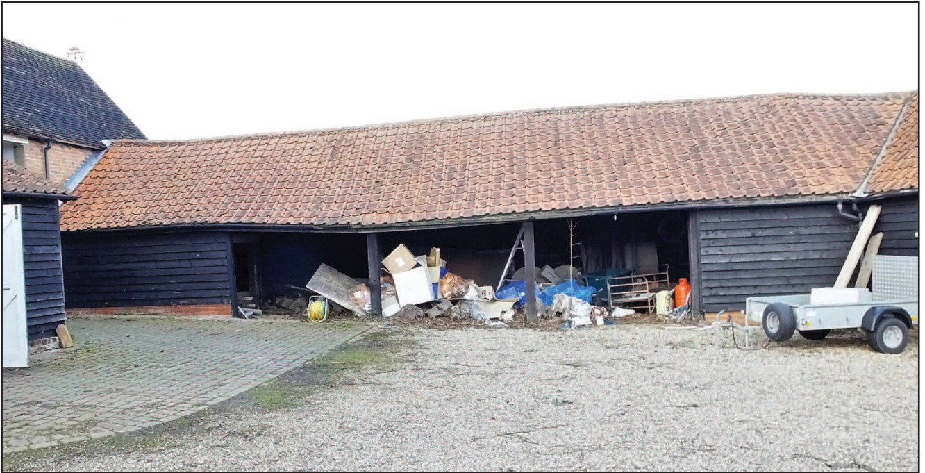
1. Cart lodge range with boarded front to two outer bays. Roofed in single Roman profile clay tiles. The existing build was totally twentieth century but left clues at each end and in the floor. (Authors photograph)
