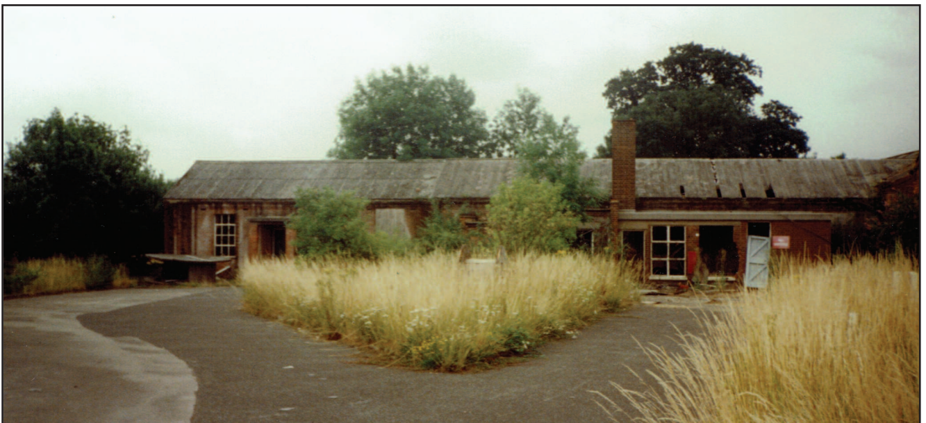
7. A view of the main building looking south at the main entrance and boiler house. (Author photograph, July 1996)
