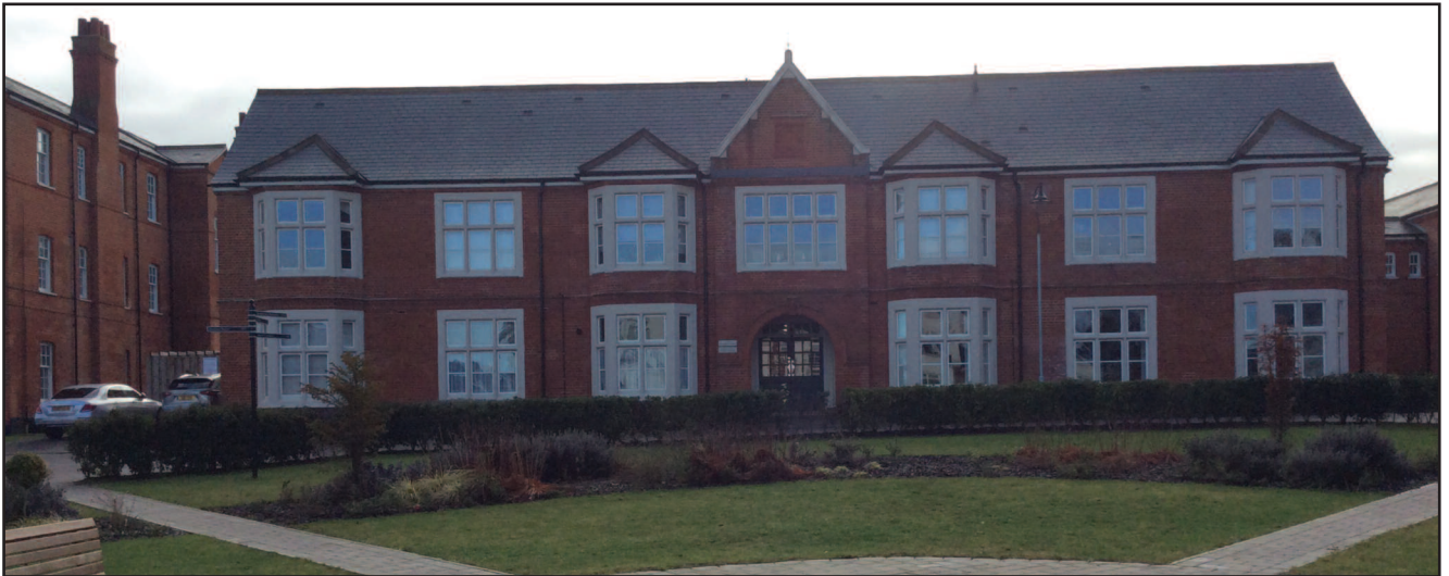
2. The renovated administration block of Chelmsford Union Workhouse, 2017. (Author's photograph)
