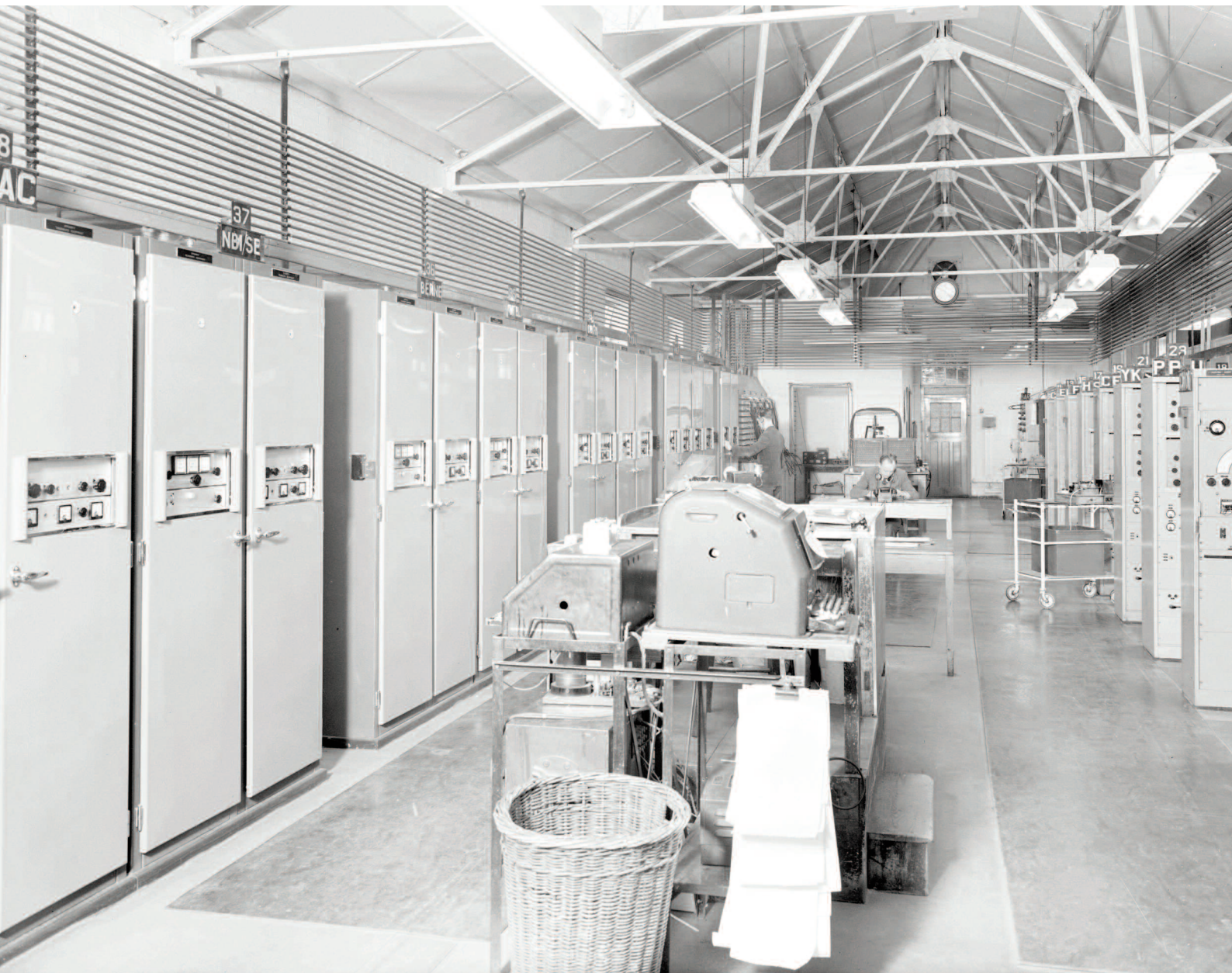
4. South Wing Marconi HR91 W/T receivers and central monitoring equipment. The wicker basket was used to collect discarded paper tape and teleprinter print-outs ready for collection and burning, c.1956. (Reproduced by courtesy of British Telecom Archives, TCB/473/P06486)
