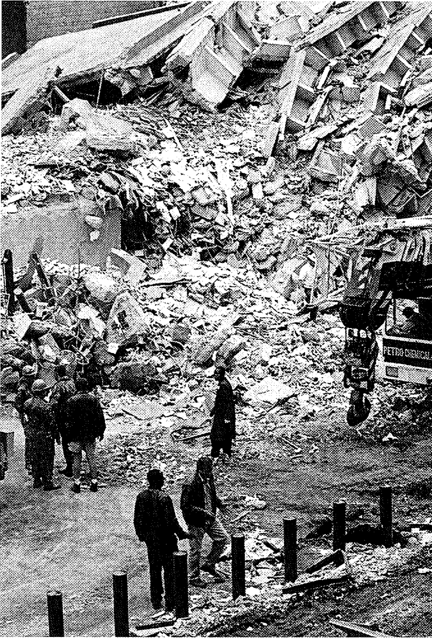
Wreckage of U.S. Embassy following bombings in downtown Nairobi, Kenya
