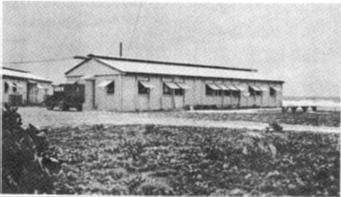
Figure 5. Typical metal buildings used at Enewetak during CASTLE.
