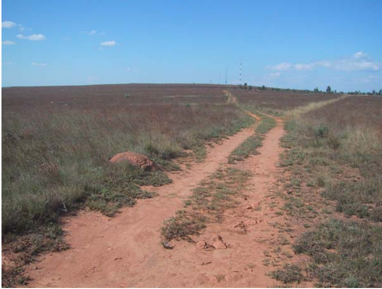
Plate 13: Upper dam access route
