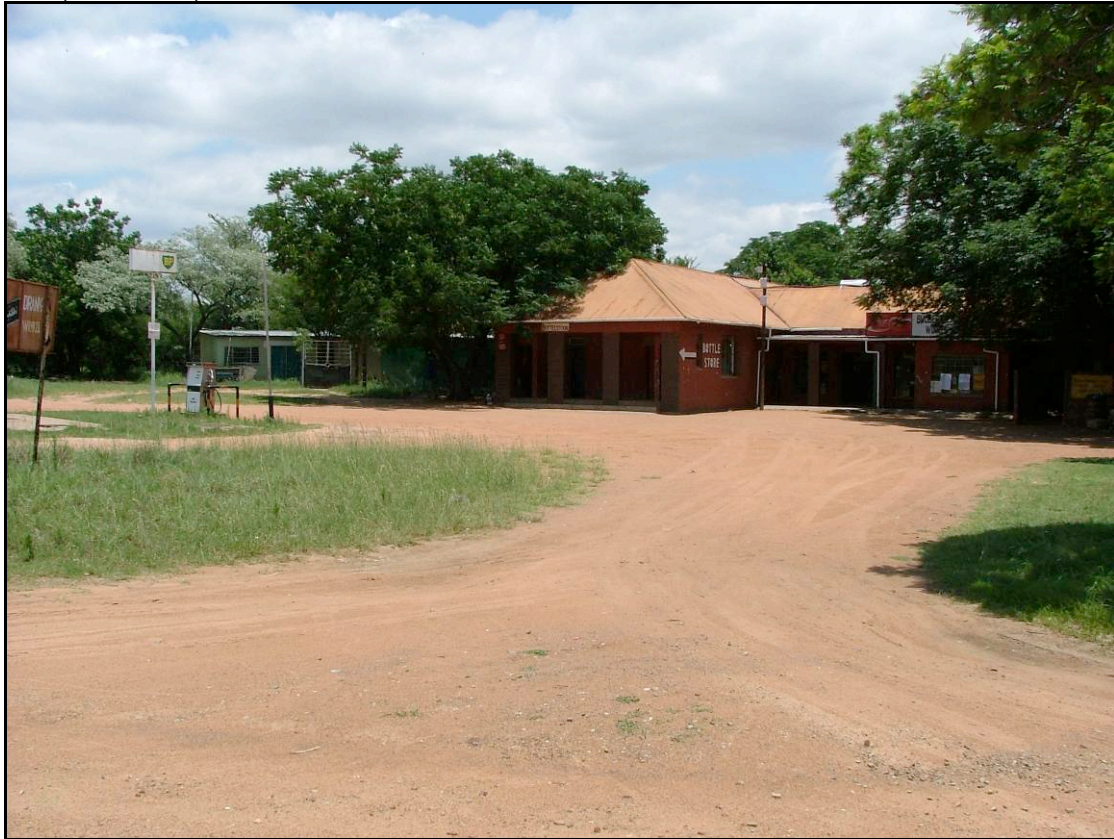
Figure 15. Bulge River shop and filling station. Just east of Bulge River Substation site (Dec.2010)
