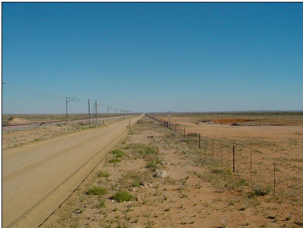
Figure 5. A southerly view along the railway line showing the adjacent service road.
