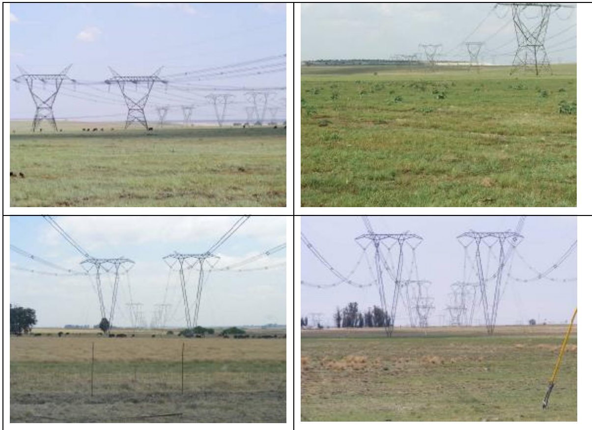
Figure 3: View of the existing power line on site
