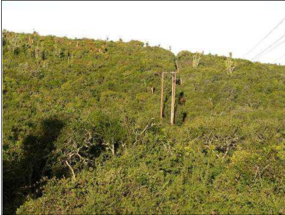
Tall Gamtoos Thicket just east of the Gamtoos River. Note location of powerlines and supports and the need to control vegetation height. Emergent tree is Euphorbia triangularis riviernaboom and grows to over 6 m tall
