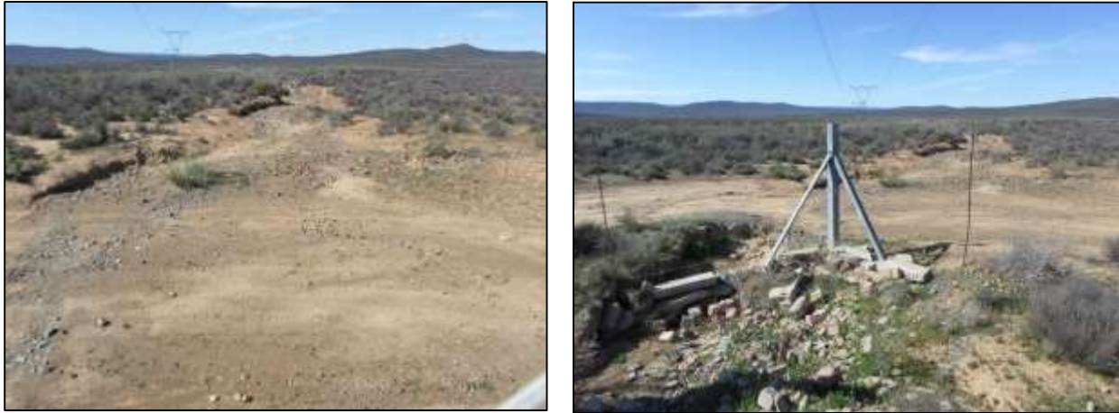
Figure 9: The section where the access road crosses the drainage line (Note the moderate levels of erosion present within this section of the drainage line).
