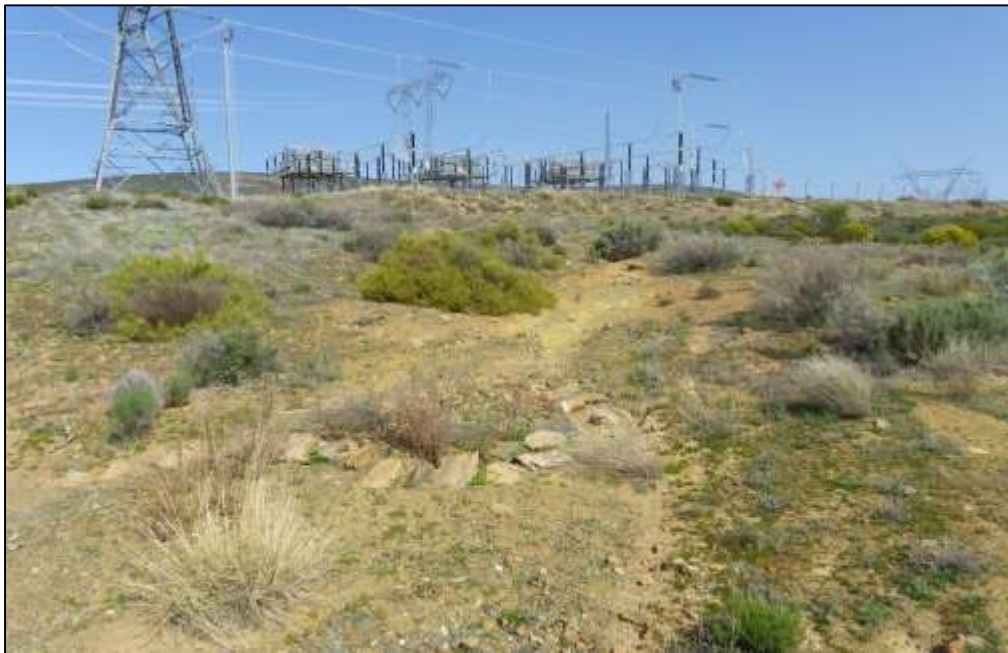
Figure 8: The species poor and highly disturbed upper section of the drainage line.
