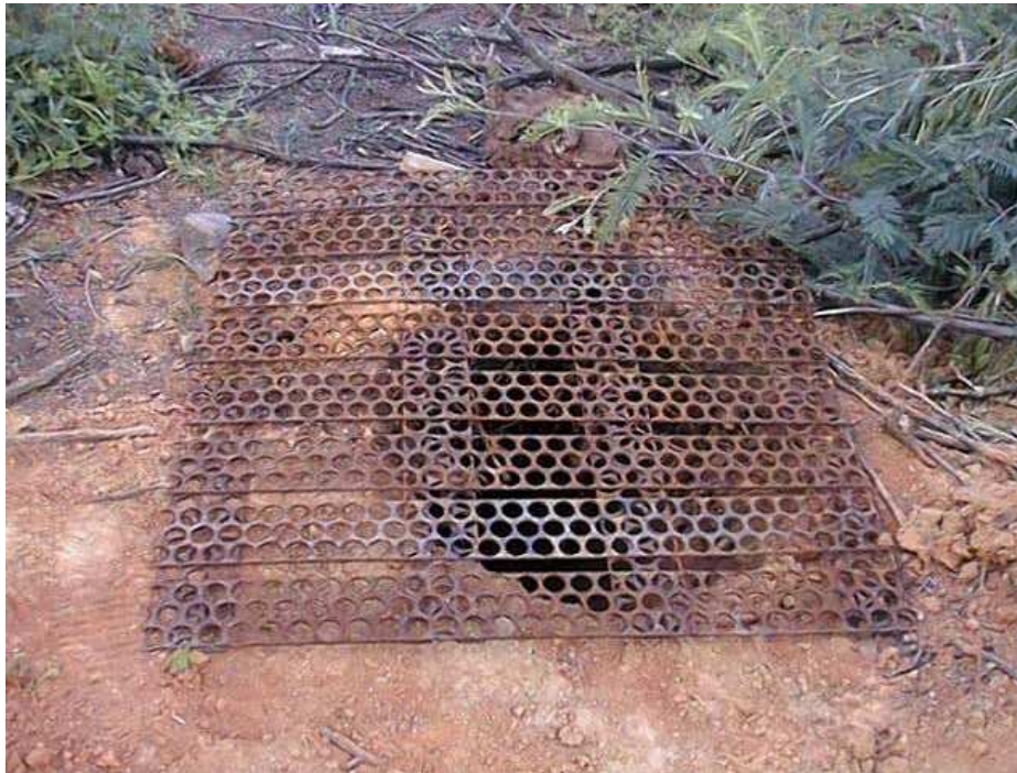
Figure 3-10: Cover over Foundations
