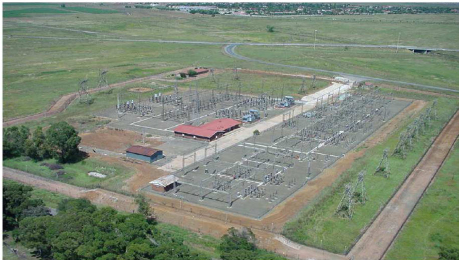
Figure 4-7: A Typical Air Insulated Substation
