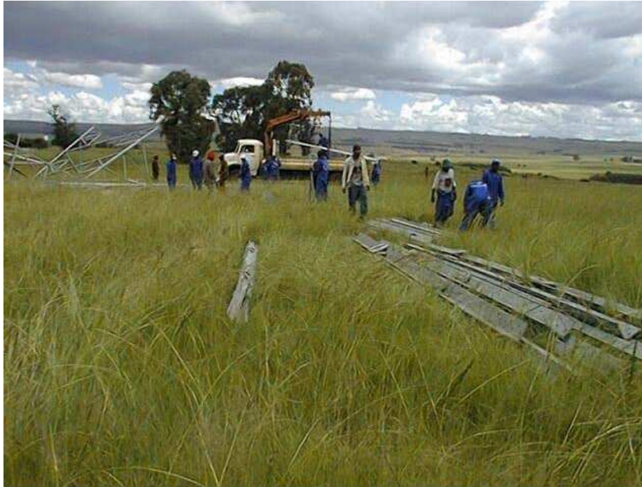
Figure 3-11: On-Site Erection of Towers
