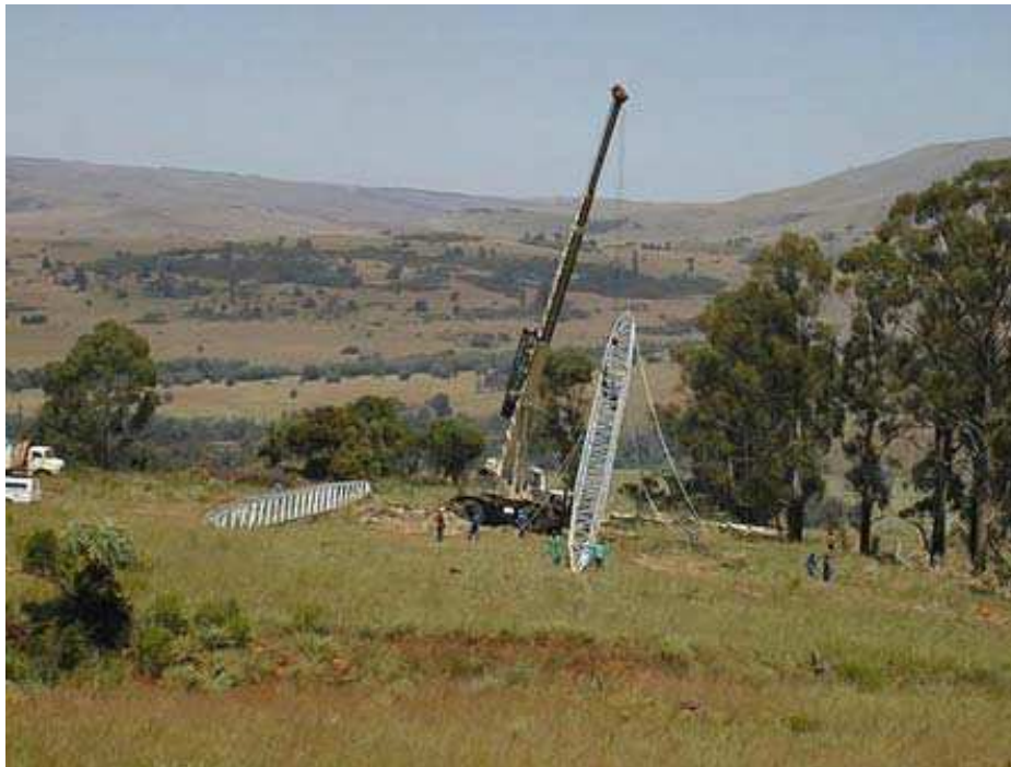
Figure 3-12: Erection of Towers by Crane
