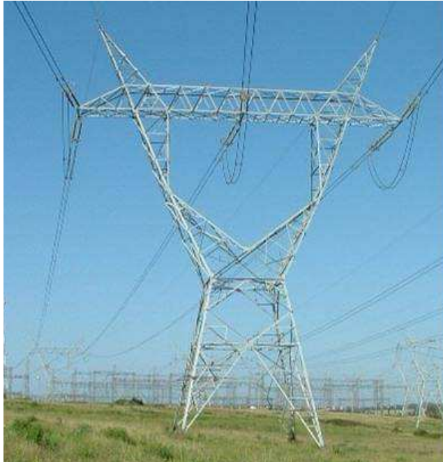
Figure 4-1: Self-supporting Tower
