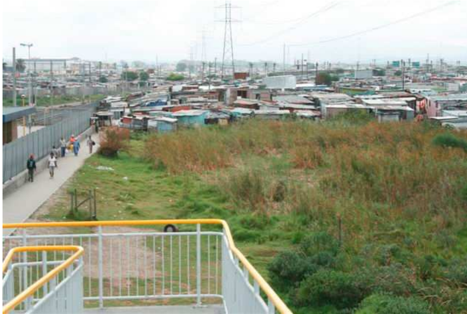
Figure 9-1: Khayelitsha Residents Living Beneath Power Lines
