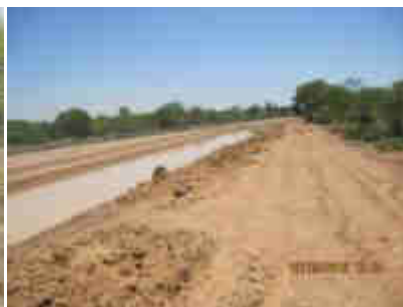
Large earthen trench around Site
