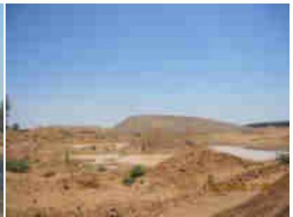
Clearing of vegetation and topsoil
