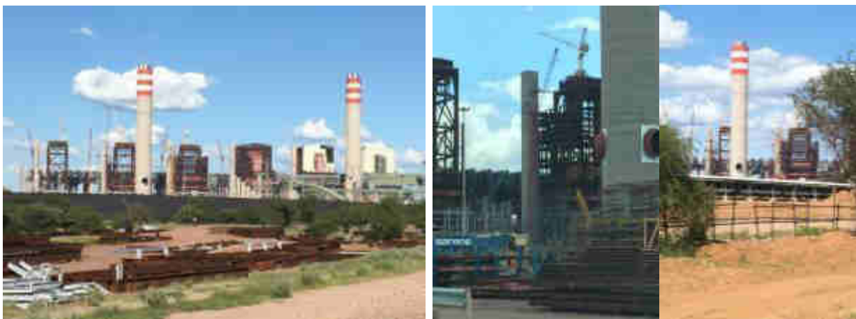
Ongoing construction of the MPS
