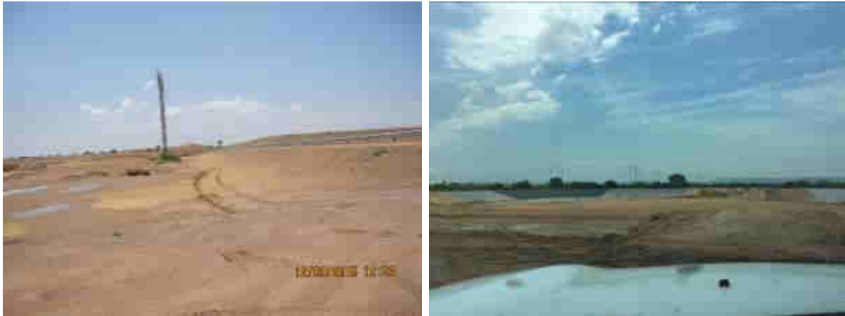
Ongoing construction of the ADF
