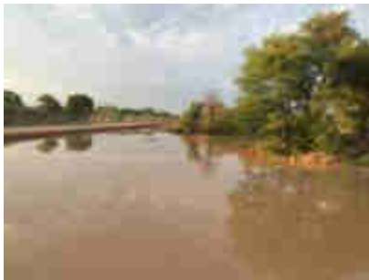
Storm water collection southern portion of the ADF
