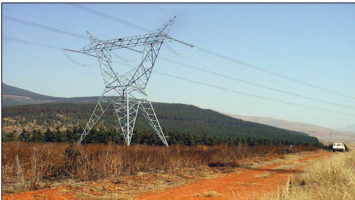
Figure 8: Guyed-V Suspension tower
