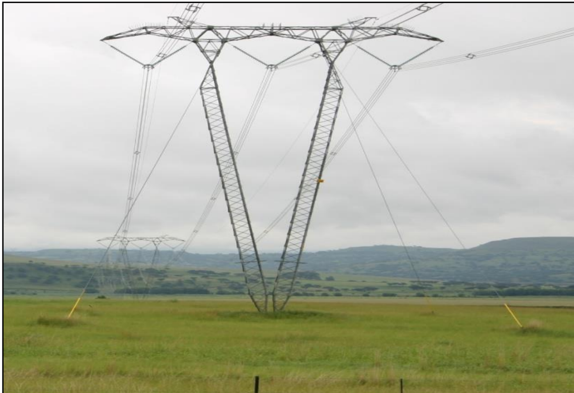
Figure 8: Guyed-V Suspension tower
