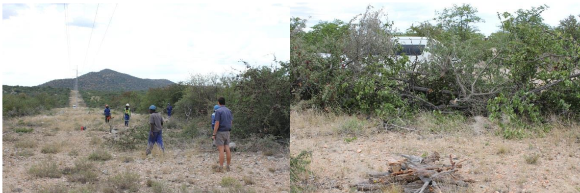
Figure 32: Maintenance team busy clearing a transmission line servitude
