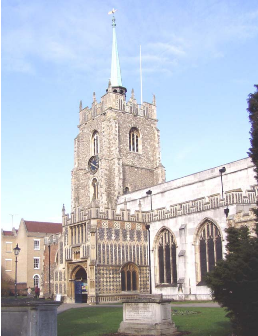
Fig: 10 Chelmsford Cathedral, showing the late 15 th century tower and flushwork decorated porch with modern buildings in the background
