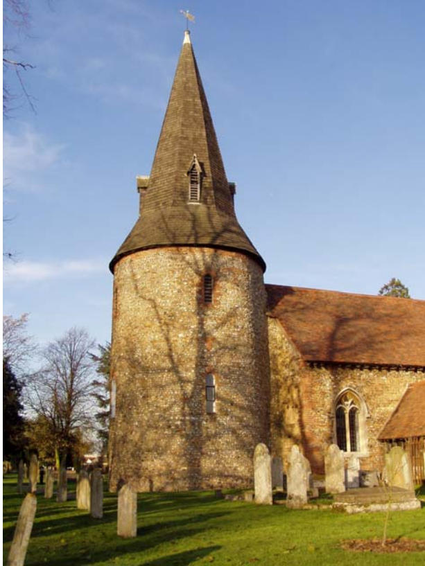
Fig: 26 Broomfield Church originally dates to the 11 th century and contains Roman brick and tile in the fabric
