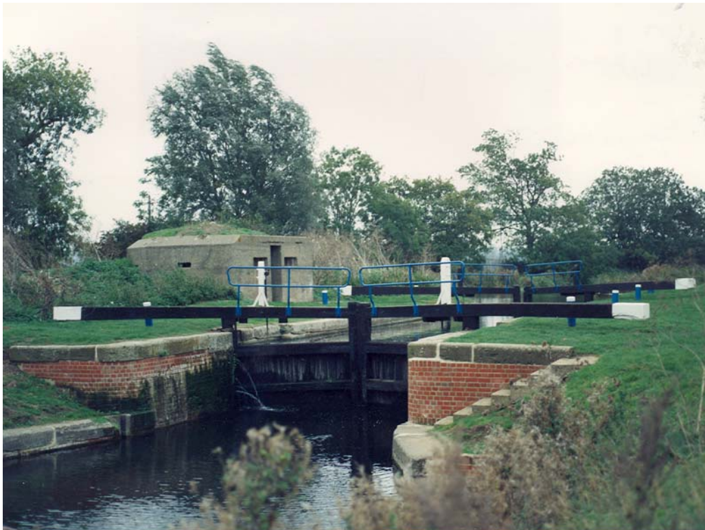
Fig: 17 Cuton Lock with a pillbox from the GHQ line in the background
